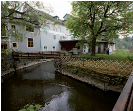
mill stream for hydroelectric power
