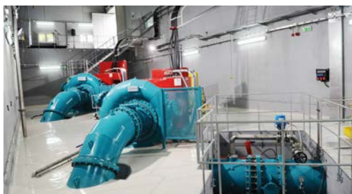
Francis Turbine HPP Zapece all pictures © GUGLER Water Turbines GmbH
