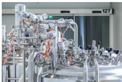
Pure Media pipe installation © Foto: Leitner
