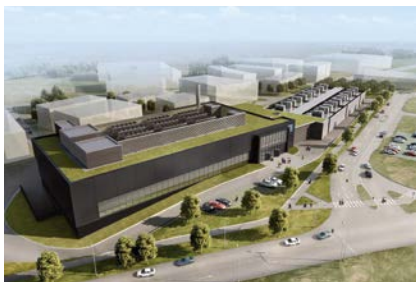
AVL turnkey solutions – early project stage
