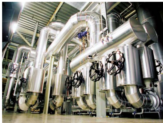
Chemical pipe installation © Foto: SMB
