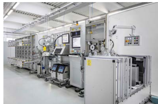
Fibre ribbon production line FRP 05 © 2018 Paul Sebesta
