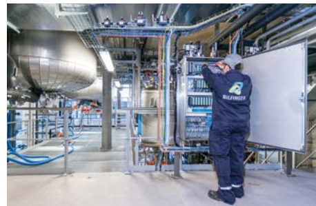
Numerous experts in automation © Bilfinger SE
