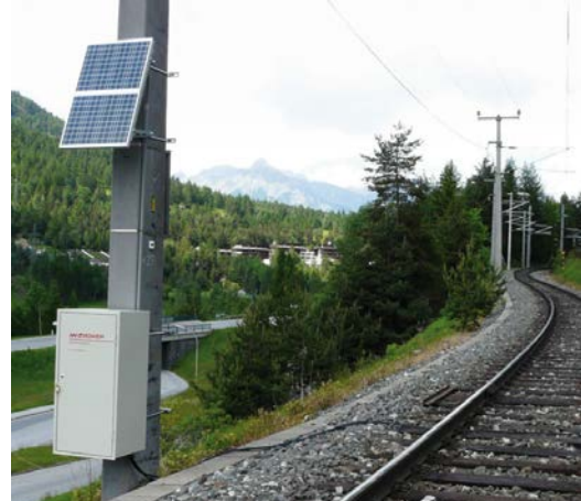
Patented rail lubrication system
