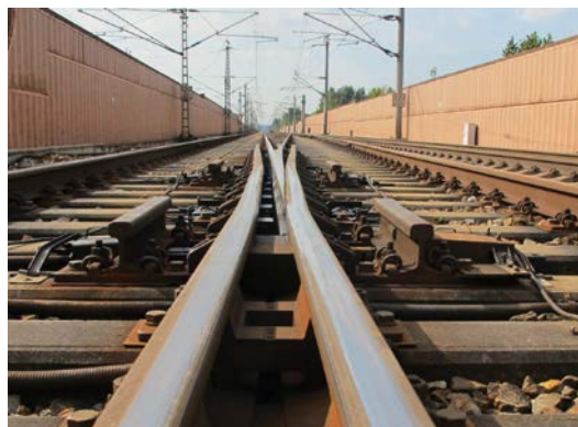
© Austroroll, HSR for swing nose crossings
