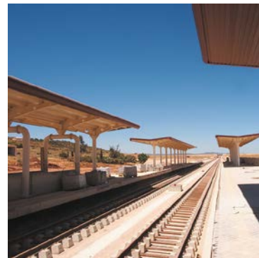
Saida railway line, Moulay-Slissen, Algeria
