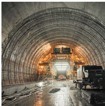
A12 Perjen Tunnel, Tyrol, Austria
