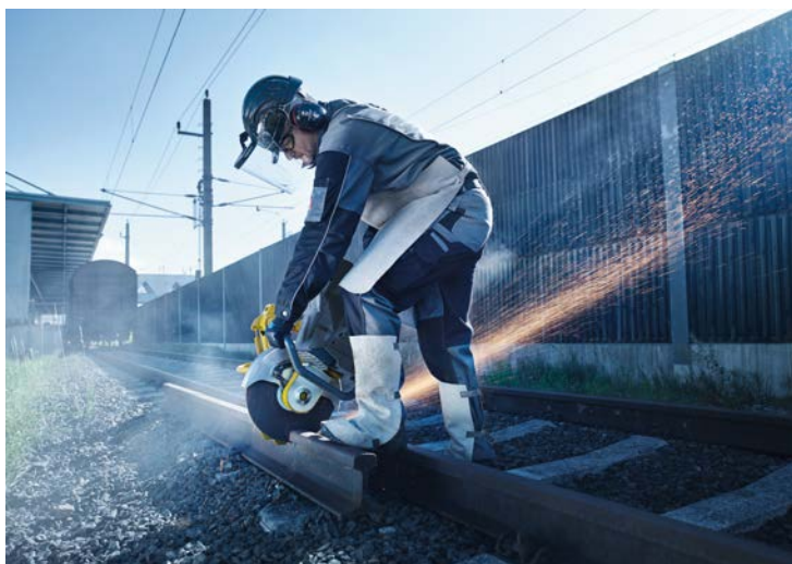
Rail cutting with TYROLIT cut-off wheel
