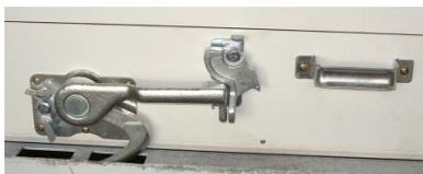
Figure 9.6 Roller shutter lock
