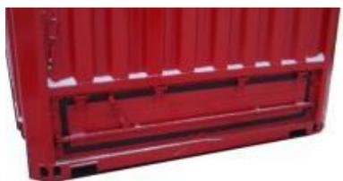
Figure 3.43 – Letterbox type hatch in container front wall
